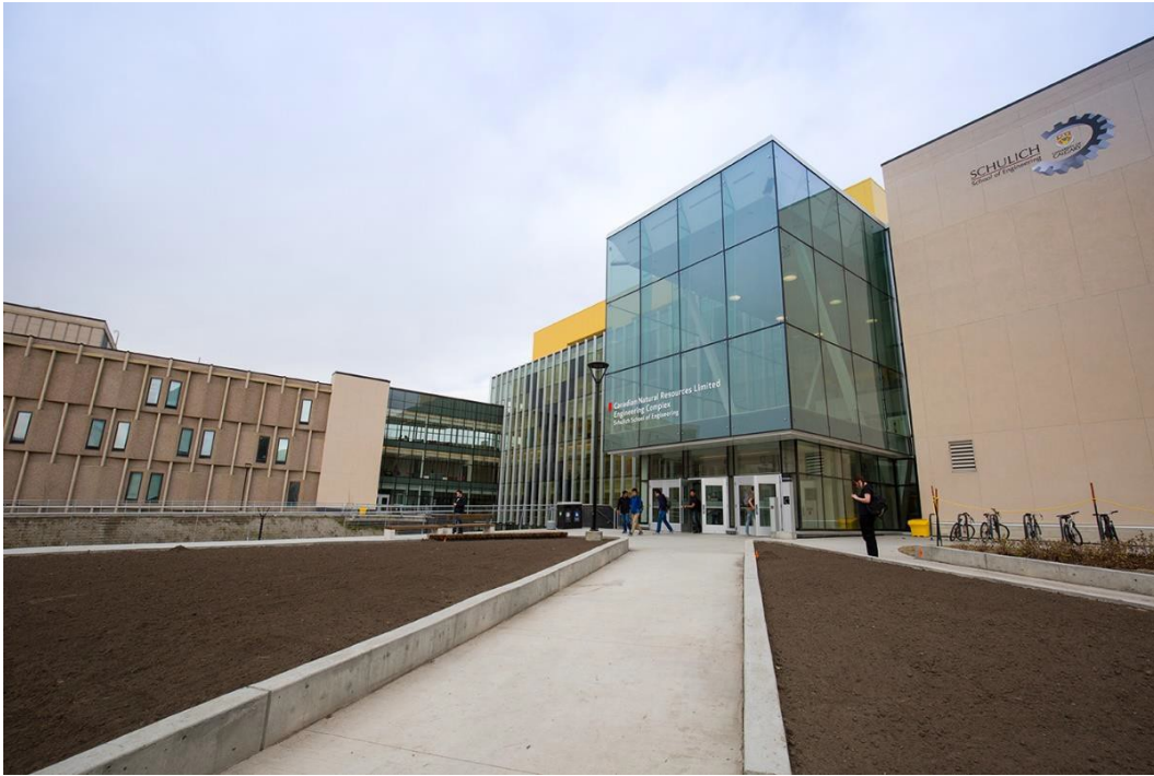
Figure 7. Canadian Natural Resources Limited Engineering Complex - i.e. Engineering Block G
