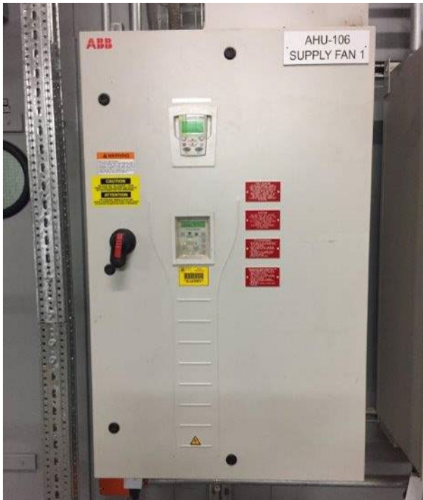
Example 49. ABB VFD
