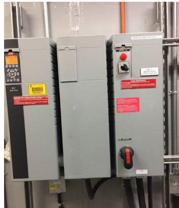
Example 48. Danfoss VFD
