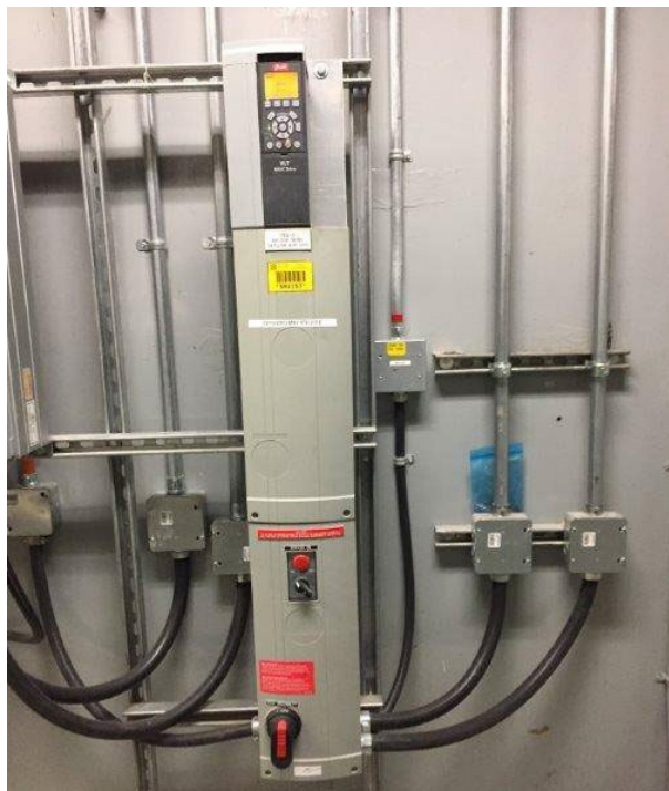
Example 47. Danfoss VFD
