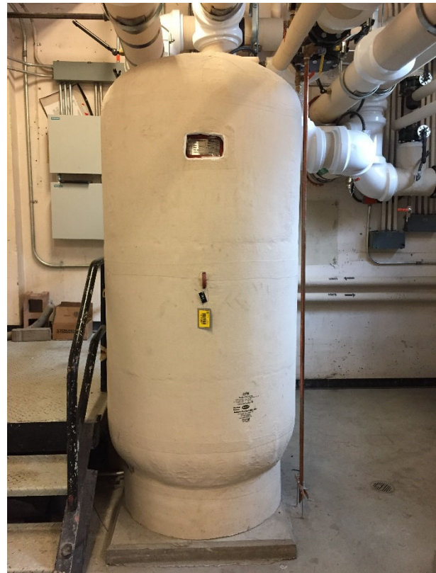
Example 14. Water Storage Tank
