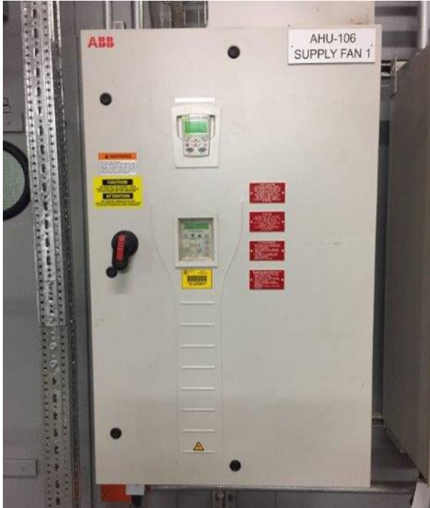
Example 49. ABB VFD
