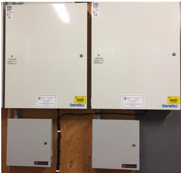
Example 31. Door Access Panels
