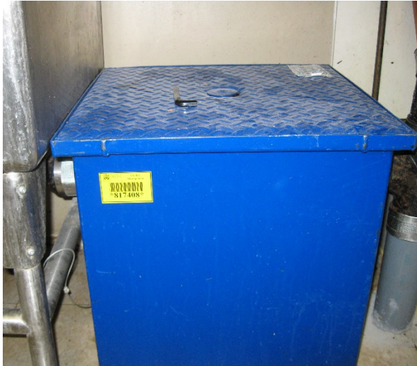
Example 9. Grease Interceptor
